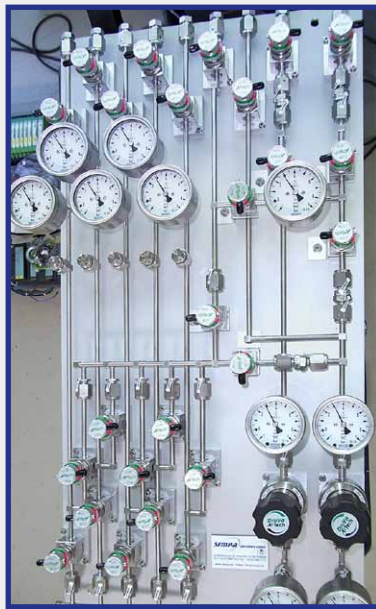
Dopant gas mixing station › Highly stable mixing ratio
