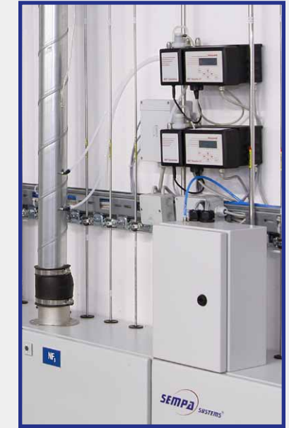
Gasdetection › Electro chemical and catalyst based GAS measurement in the ppb ... vol% range
